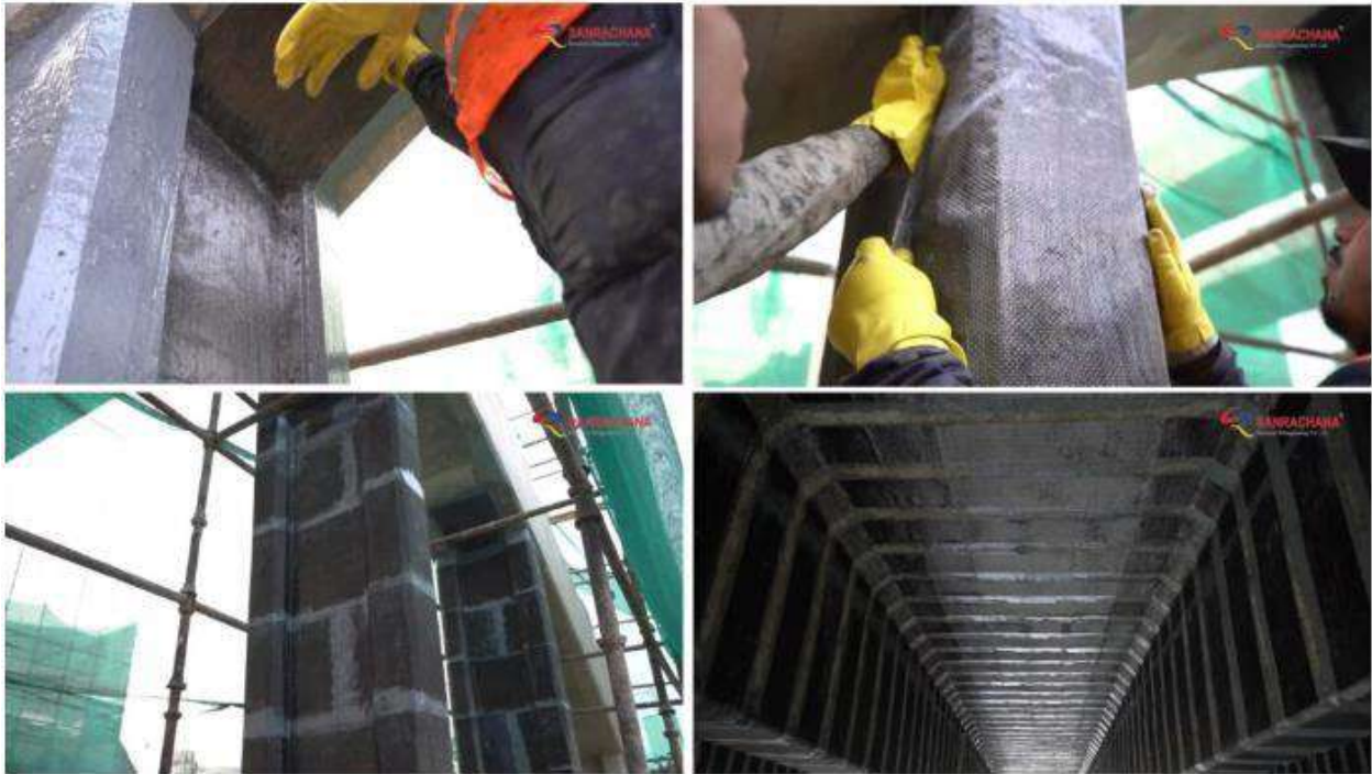
Fig. 4 Application of SRM carbon laminates & SRM C-wraps
