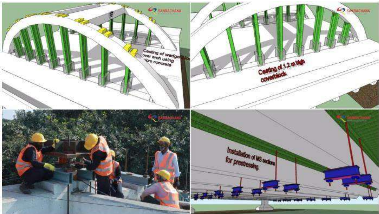
Fig. 5 Illustration of strengthening activities using MC Alloy Bars
